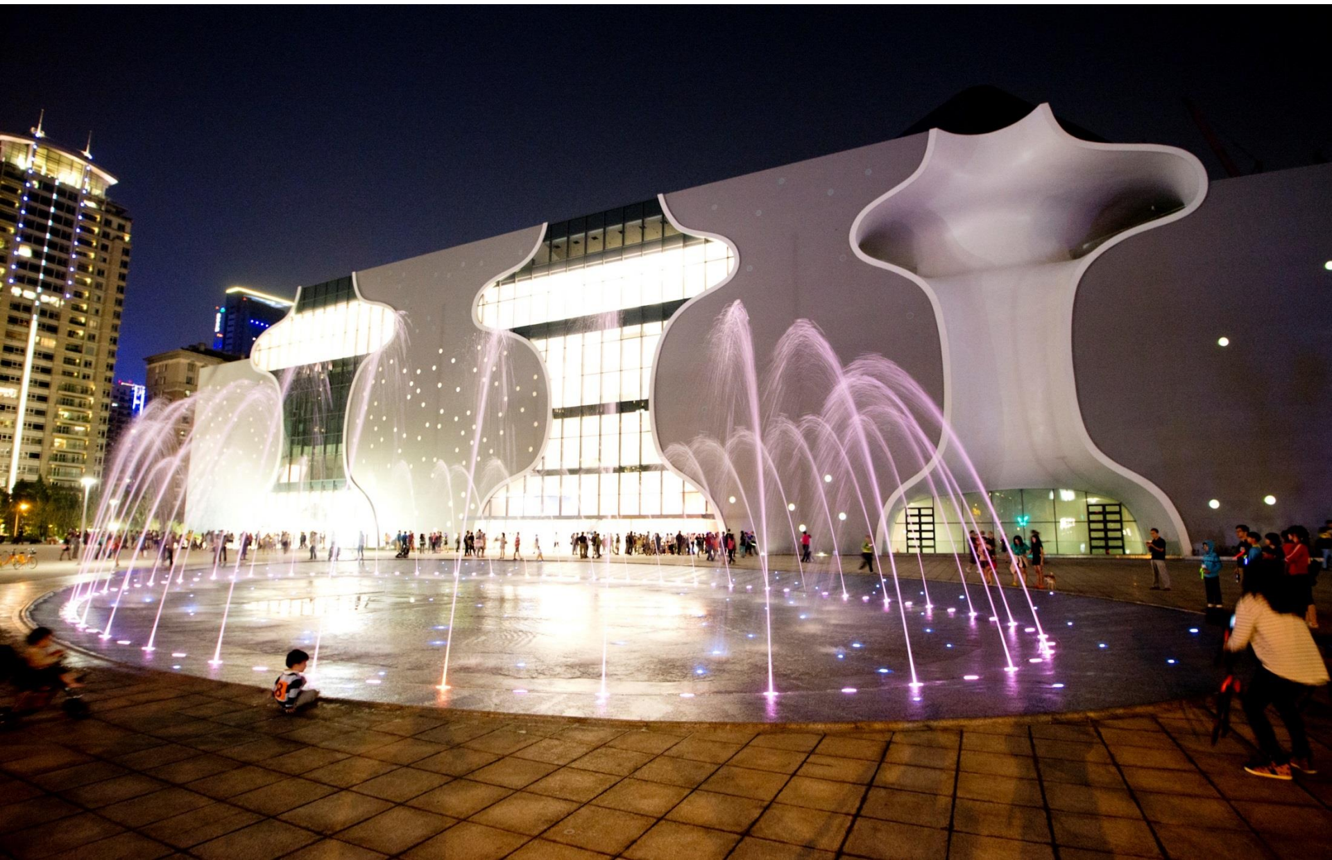
TAICHUNG OPERA HOUSE
